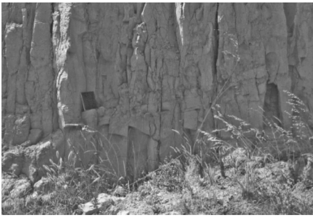
Fig. 11. Vertical jointing: outcrops in Agrio river
