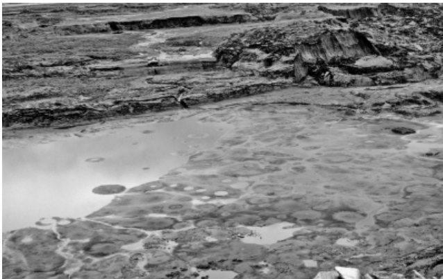
Fig. 22. Mud volcanoes observed a few hours after failure on surface of depressed basin upstream of slid dam
