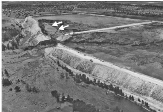
Fig. 19. The straight line, indicated by arrows, shows the position of the upstream scar of the slide
